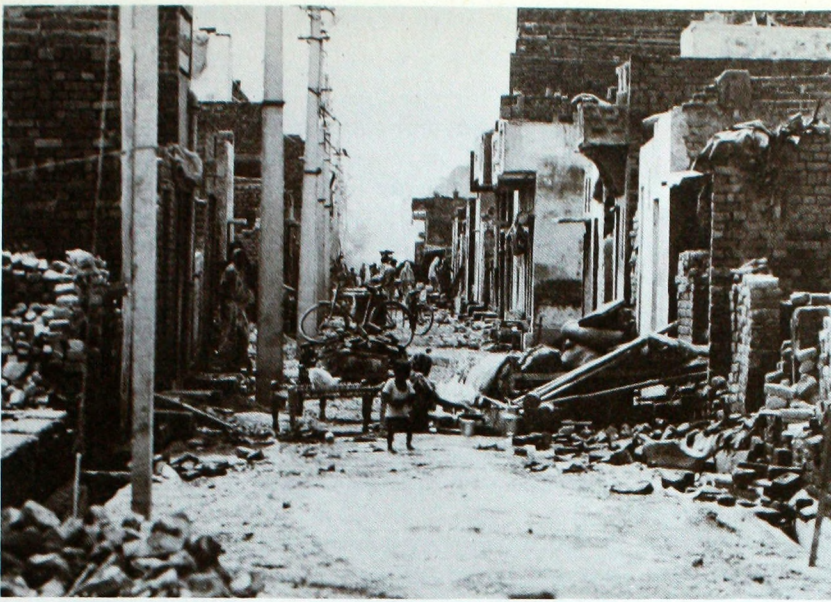
These homes in a suburb of New Delhi were buried under ten feet of water for three days. The 130,000 residents of the area returned from relief camps to find their homes collapsed, their property looted, and mud covering everything.
